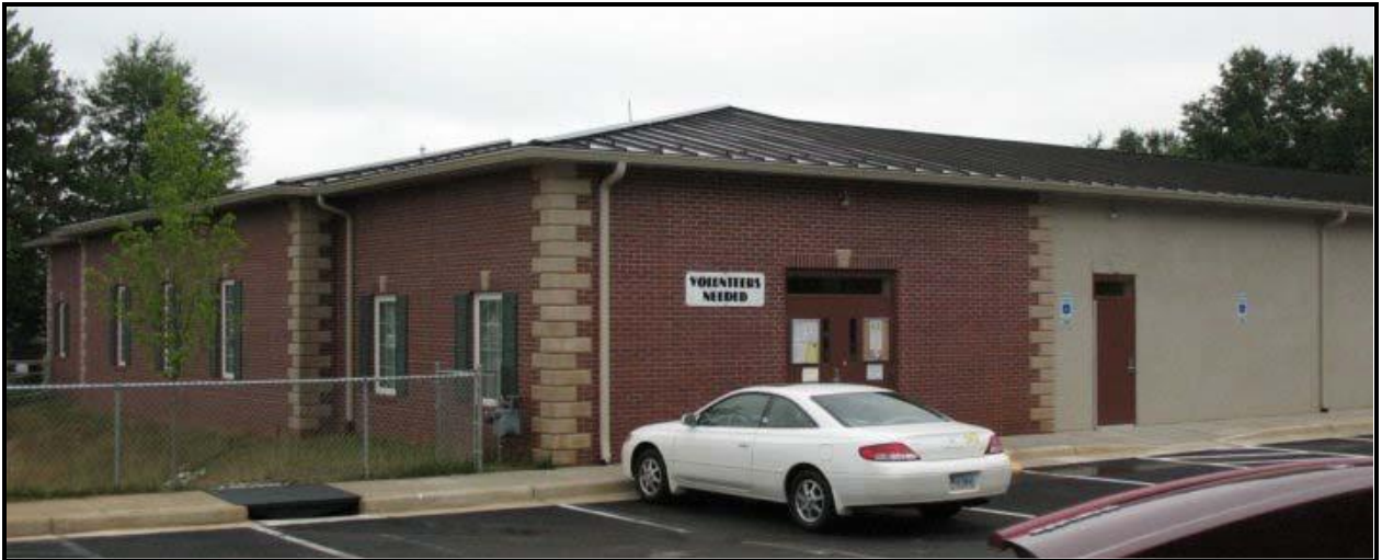
Front and west side view of building addition
