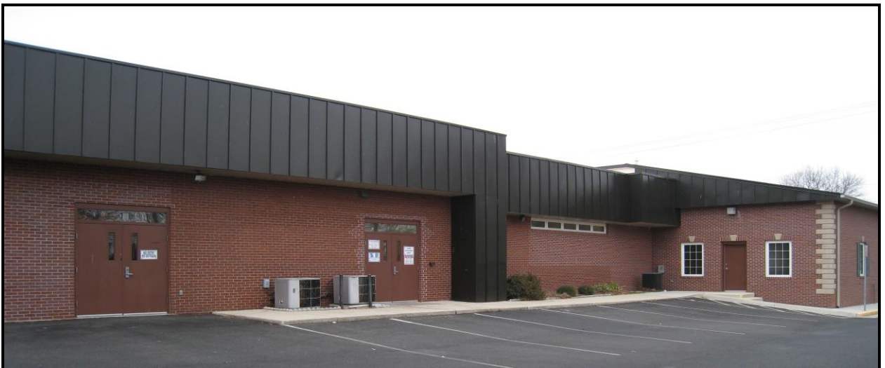
East side view of building addition
